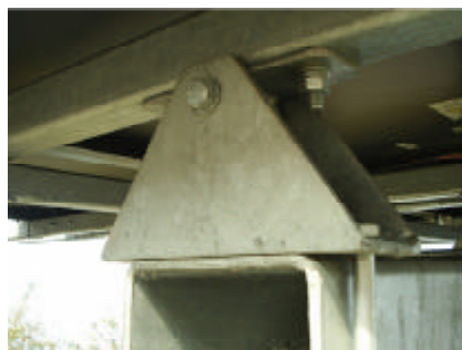
Hinges of the tracked frame
